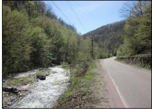
Figure 4. Rehabilitation of the communal road DC 286 between the localities Băița and Băița Plai an investment made through the Romanian Agency for Sustainable Development of Industrial Areas (ARDDZI)
