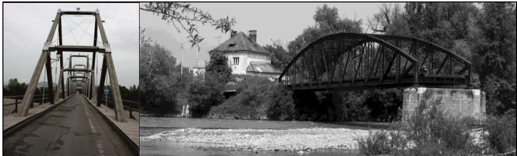
Figure 7. Wooden historical bridge between Sighetu-Marmăției (Romania) and Solotvino (Ukraine) – left; The rest of historical iron bridge between Teacev (Ukraine) and Teceu Mic (Romania) – right (Photo: A. Ilieș)
