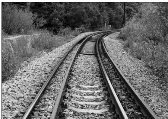
Figure 5. Double railway in Maramureş area (normal-European and large-Ukrainian ex-soviet) (Photo: A. Ilieş)
