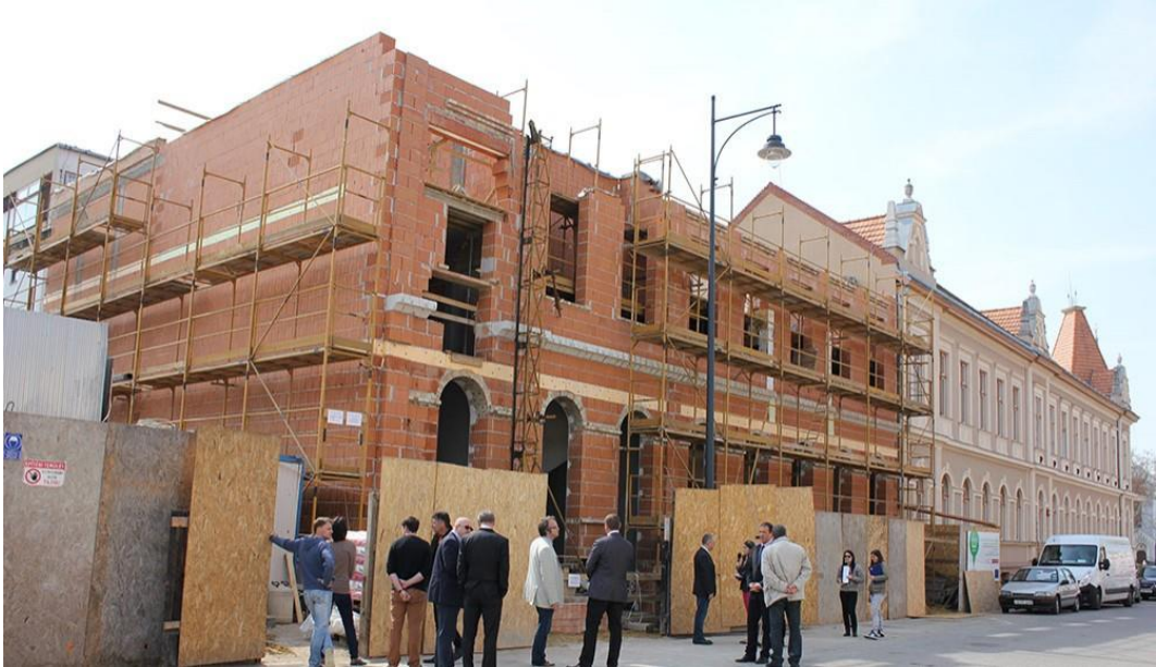
Photo 4 The Petöfi Street wing of the Hajdúböszörmény District Office (investment has been already finished) (Source: news.hajduboszormeny.hu)
