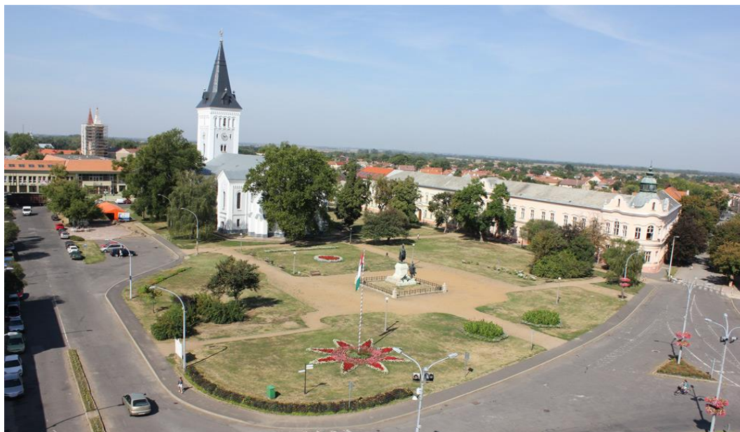
Photo 1. The condition of Bocskai Square before the renovation (photograph from the eastern side) (Source: www.hbapro.hu)
